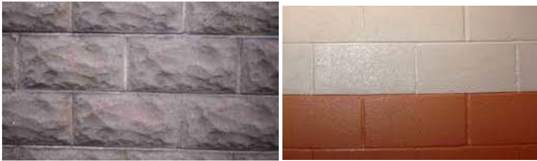
Figure 2 Finished concrete block is acceptable.
