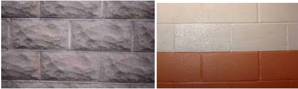
Figure 2. Finished concrete block is acceptable.
